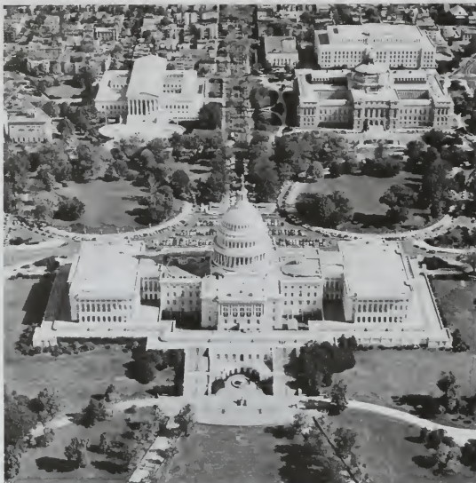
Capitol Hill, with the Capitol in the foreground. The Senate occupies the left wing and the House of Representatives the right. The Supreme Court is at upper left and buildings of the Library of Congress at upper right.
